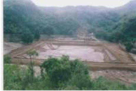
Sarasvati River Sarovar, under construction, at Adi Badri (June 2004)
